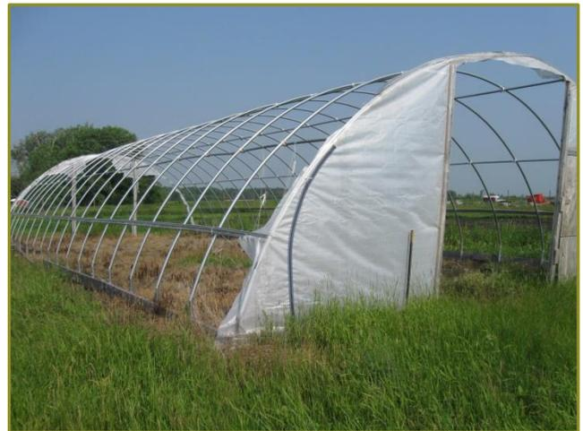
Fig. 1: Weather torn high tunnel
